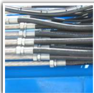
HYDRAULIC STAINLESS STEEL PIPING
