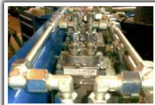
HYDRAULIC DISTRIBUTORS WITH SAFETY VALVES
