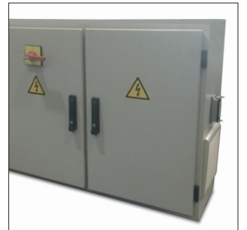
9 Crane control panel
