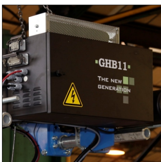
17 Hoist electric cabinet
